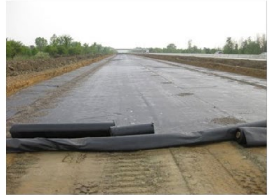
I-94 St. Clair and Macomb Counties, Michigan, woven geotextile separator on subgrade
